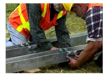
7. For hinge assembly, place the upper and lower post sections together on a flat level surface. Place the hinge plates on the outer surface of the post and install and tighten bolts.
