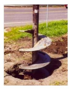
3. Auger the hole for the foundation and position reinforcing.
