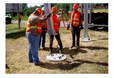
11. Suspend the post assembly above the post foundation and insert the special bolts through the holes in the bracket and thread them snugly into the couplings.
